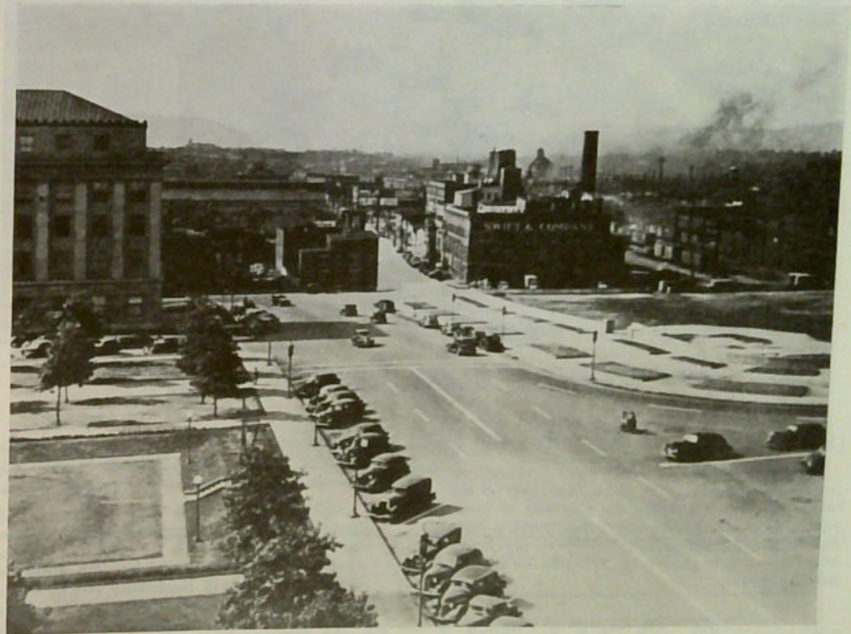
Fig. 12. The present offset intersection of Fisher Plaza, Seventh and North Streets, forms a traffic hazard.
