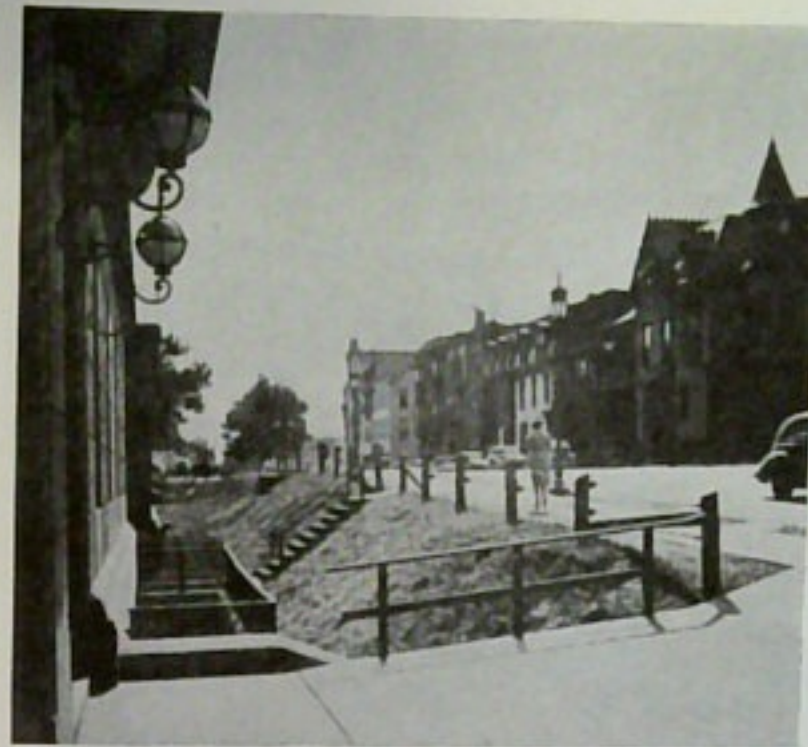
Fig. 9. The ungraded hump at Sixth and North Streets still persists, eleven years after completion of the North Office Building, to the main entrance of which a plank bridge serves as the approach.
